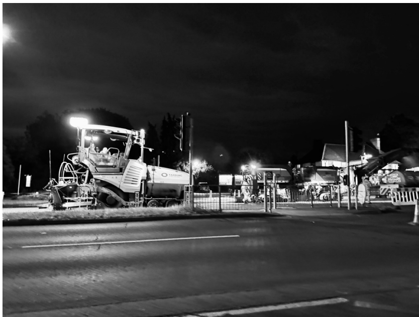
Image 1. Night workers in the construction sector (Image Didobi)
